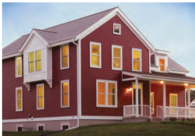
Figure 4.5 (PP): The PATH Concept House designed by Torti Gallas and Partners features a 75-year exterior shell with insulated vinyl siding. This LEED-Silver-certified home won the NAHB 2008 Green/Sustainable Project Award.
