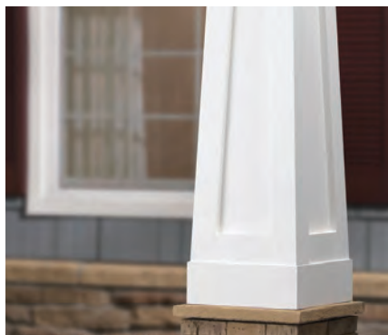
Figure 4.2 (PP): A tapered post constructed with cellular PVC.
