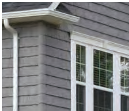
Figure 4.3 (PP): A mitered corner using polypropylene shake.
