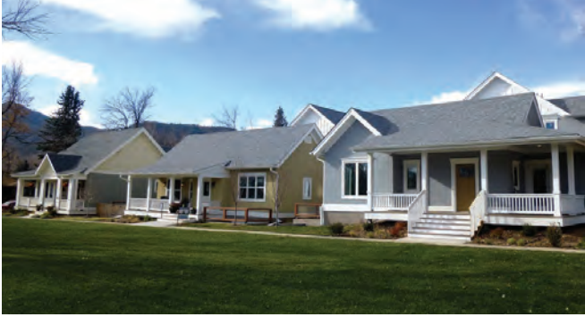
Figure 3.20: Generously sized porches facing a pocket park. Porches can create a relatable human scale for the block face and a comfortable walking environment on the sidewalk.
