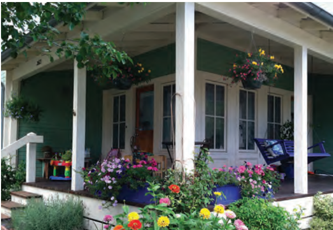
Figure 3.25: Exposed rafters and simple column and beam details create a pleasant porch with interesting textures.
