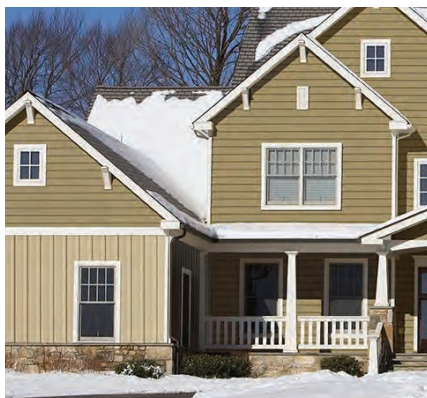
Figure 4.15 (PP): An example for the use of vertical vinyl siding as accent.
