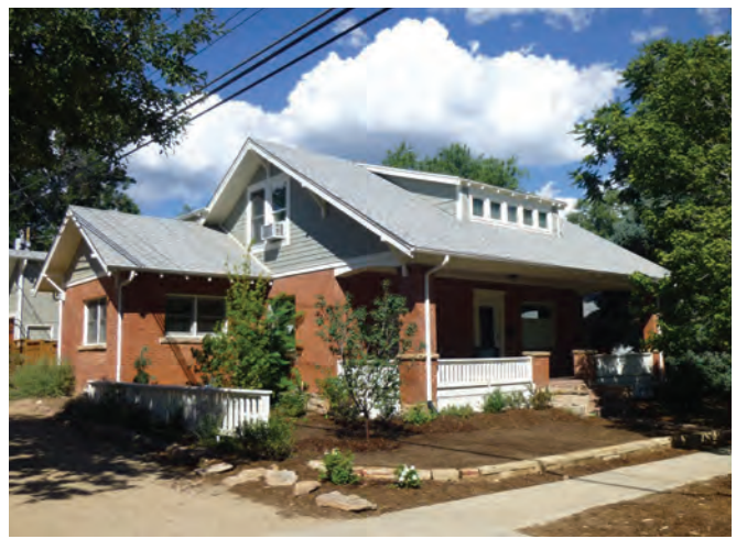
Figures 2.10, 2.11, 2.12, and 2.13: Four buildings in Craftsman style present a single-story scale to the street. The primary roofs can be parallel to the sidewalk (upper left and lower right), perpendicular to the street (upper right), or crisscrossed (lower left). Note how the porch roofs are an integral part of the primary roof geometry. Large overhangs, brackets, and window trims express a balanced Craftsman style. On the lower right is a one-and-a-half-story building with a shed dormer.
