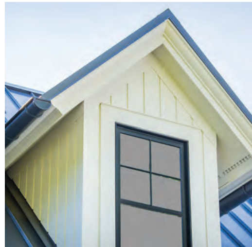
Figure 3.13 (PP): A dormer demonstrates traditional detailing: Eaves project in the direction of the roof pitch, and the rake projects forward. An ornated molding is incorporated into the trim work at the rake and echoes the subtle curves of the half-round gutters.
