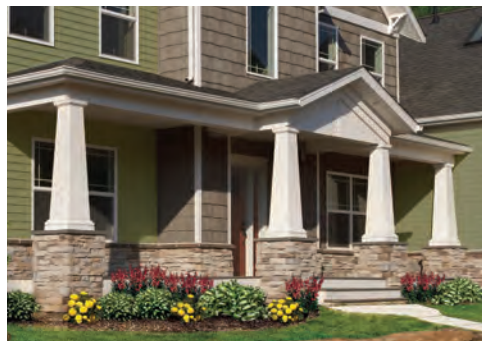
Figures 3.22, 3.23 (PP), and 3.24 (PP): Three examples of amply-sized porches that express the character of their architectural styles. The primary elements to consider are column sizes, bases, and capitals.
