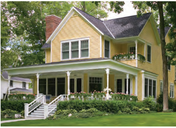
Figures 3.3 and 3.4: A comparison of two buildings that emphasize the importance of creating a legible hierarchy of primary, secondary, and tertiary forms in designing a well-articulated façade. The example on the left (PP) has a simple forward-facing gable (the primary form) with a porch (the secondary form) added and a balcony subtracted on the second floor. The example on the right (PP), on the other hand, employs five forward-facing gables that are competing, making the whole composition too crowded.
