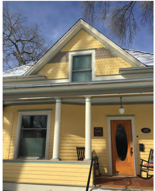
Figure 3.53 (PP): A historic landmark building with horizontal siding in the East Side Historic District, Longmont, Colorado. Note the dormer-face shakes are a polymeric product.
