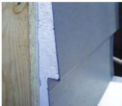
Figure 4.9 (PP): Insulated siding presents a flat profile, without the convex shape of traditional vinyl clapboard.
