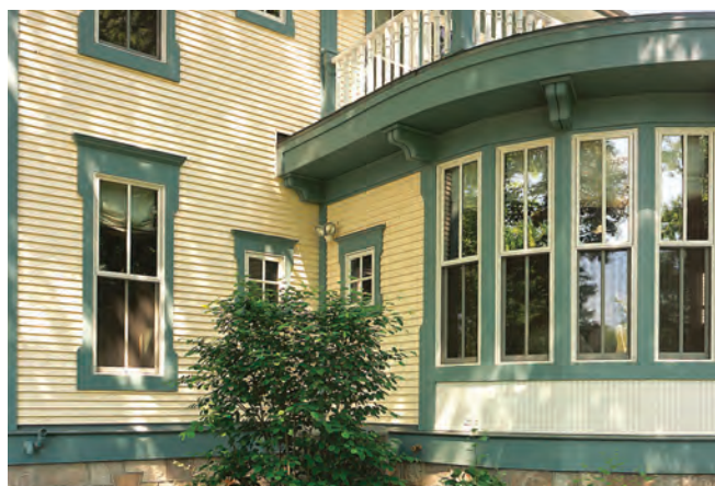
Figure 4.1 (PP): A corner of an ornate Italianate building with trims and embellishments in polymeric materials.
