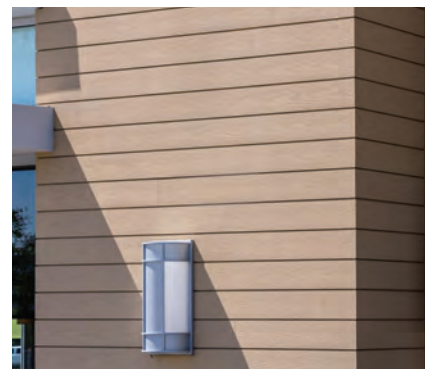
Figure 4.4 (PP): A mitered corner using Polyash siding.
