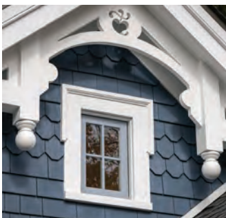
Figures 3.35 (PP), 3.36 (PP), 3.37 (PP), and 3.38 (PP): Various trims and embellishments can include ornate gable-end pediments, porch-column brackets, ornate columns, balustrades, and window trims (all examples are polymeric products).
