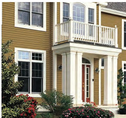
Figure 4.16 (PP): A building employing cellular PVC trims and insulated siding.
