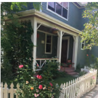
Figures 3.22, 3.23 (PP), and 3.24 (PP): Three examples of amply-sized porches that express the character of their architectural styles. The primary elements to consider are column sizes, bases, and capitals.
