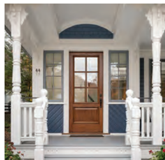
Figures 3.35 (PP), 3.36 (PP), 3.37 (PP), and 3.38 (PP): Various trims and embellishments can include ornate gable-end pediments, porch-column brackets, ornate columns, balustrades, and window trims (all examples are polymeric products).
