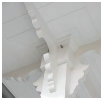
Figures 3.35 (PP), 3.36 (PP), 3.37 (PP), and 3.38 (PP): Various trims and embellishments can include ornate gable-end pediments, porch-column brackets, ornate columns, balustrades, and window trims (all examples are polymeric products).
