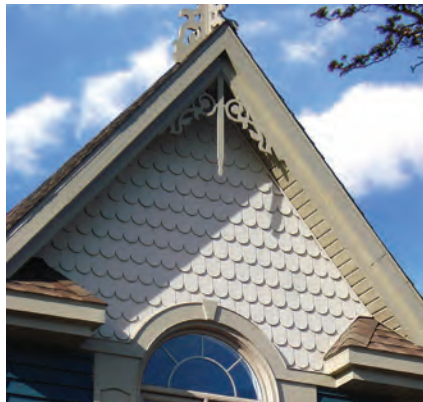
Figure 4.13 (PP): Vinyl shingle shapes on a historic house.
