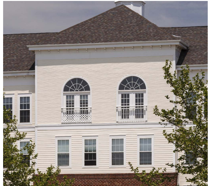
Figure 52: Apartments at Lakelands, Gaithersburg, MD, by DPZ CoDesign with vinyl clapboard siding, vented vinyl soffits, and cellular PVC trims, columns, and embellishments.
