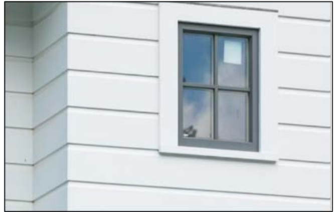
Figure 95: A tooled mitered corner in polyash.
