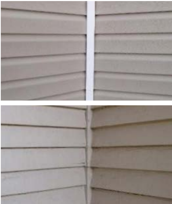
Figures 100 & 101: At top, standard vinyl inside trim; at bottom, traditional wood inside trim. Specify inside corner trim with the same color as the siding.
