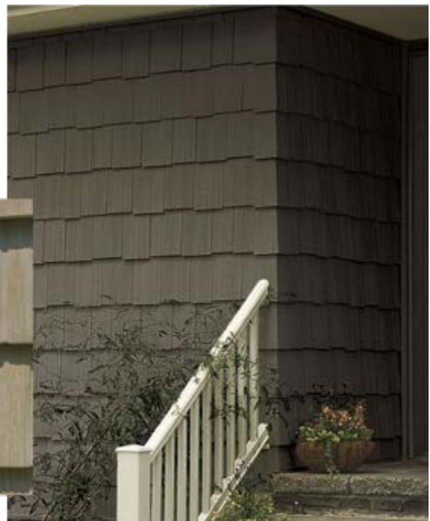
Figure 96: Mitered corner in cellular PVC shake.
