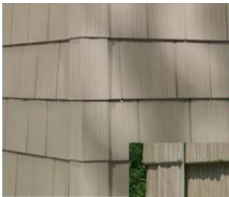
Figure 94 (i-94): Vinyl outside corner post with a simple but elegant profile.
