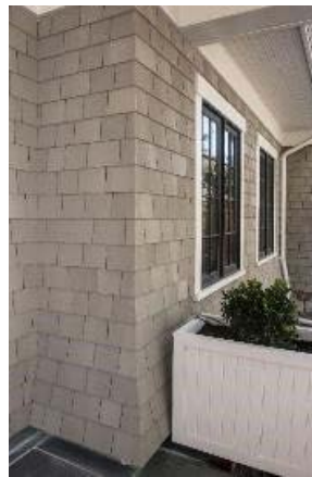
Figure 96: Mitered corner in cellular PVC shake.
