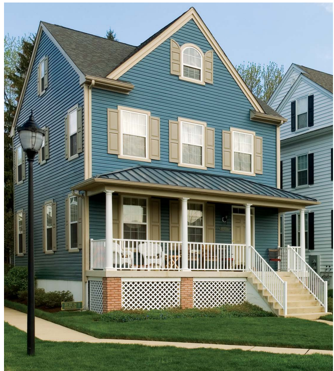
Figure 10: Example of horizontal Dutch lap vinyl siding at Lantern Hill, Doylestown, PA, designed by Torti Gallas + Partners.
