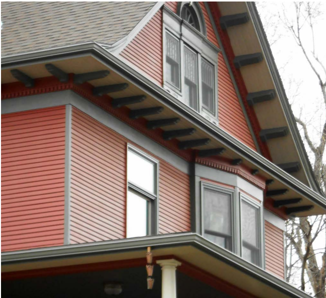
Figure 51: Italianate house in Lincoln, NE, with vinyl clapboard siding and vinyl band below eaves.
