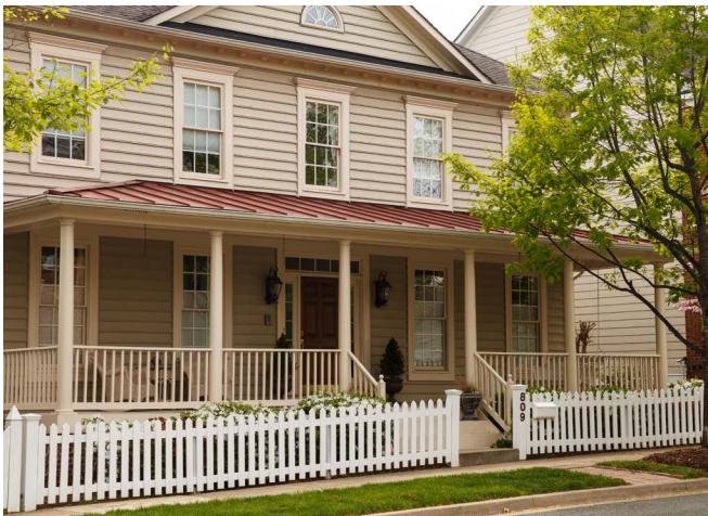
Figure 9: Example of horizontal beaded vinyl siding at the Lakelands Neighborhood, Gaithersburg, MD, by DPZ CoDesign.
