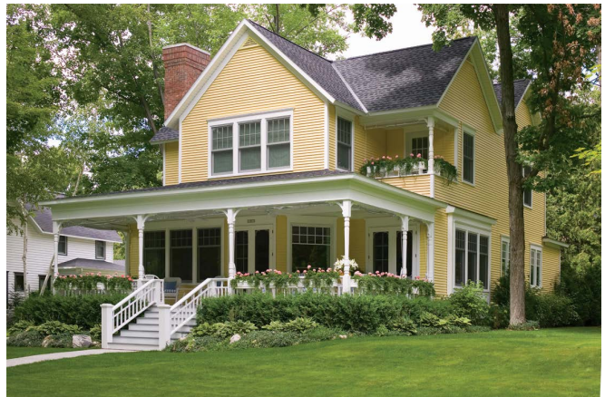
Figure 1: Polymeric claddings and trim come in sufficient varieties and colors to clad many traditional building styles, such as this Folk Victorian home. The columns and trims in the photo are cellular PVC while the siding is vinyl clapboard.
