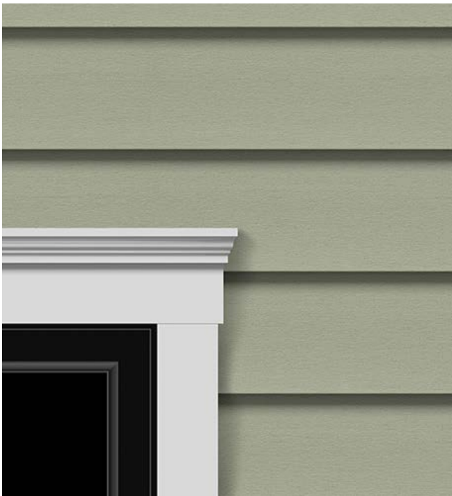
Figure 81: Cellular PVC trims with built-in J-channel (rabbeted pocket for receiving siding) may still appear too thin for a realistic perspective from the side.
