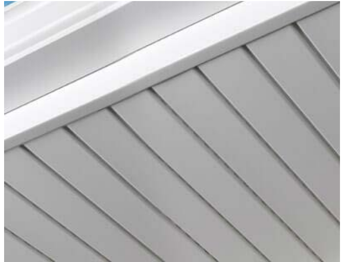
Figure 106: Look carefully and the perforations in the grooves of this premium vinyl soffit are just visible.
