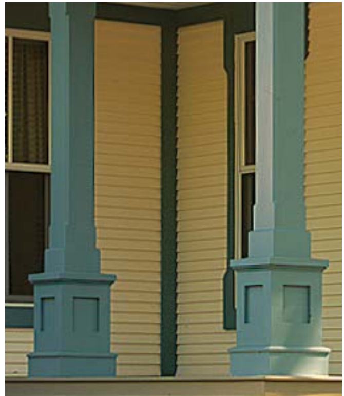
Figure 102: A wide lineal installed vertically can create a handsome inside corner post.
