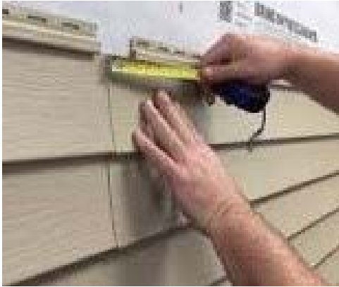
Figure 85: Single panel of siding includes two-panel profiles so that the end laps create the illusion of stacked seams.
