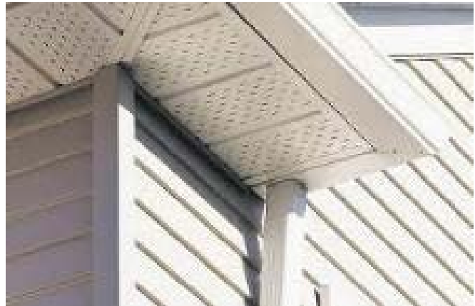
Figure 107: Perforated vinyl soffit.
