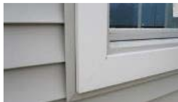
Figure 78: When J-channel matches the siding color, it adds a termination uncharacteristic of wood siding.
