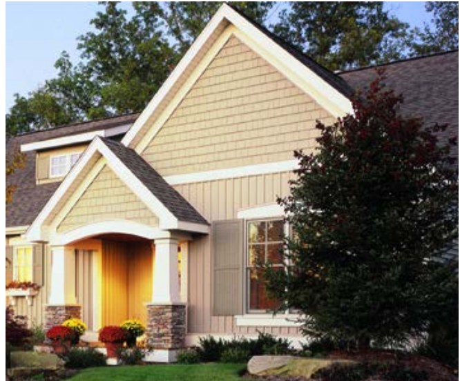
Figure 91: A typical transition between siding on the body of the house, in this case board-and-batten, and another siding on the gable end, in this case vinyl shake. The transition is mediated by a horizontal band. To ensure continuous drainage and material attachment to the structure, the installer must use the correct functional trim.
