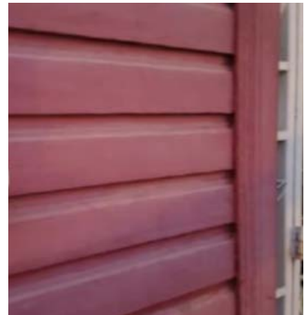
Figure 89: The shadow line on wood siding is similar to the Dutch lap in vinyl.
