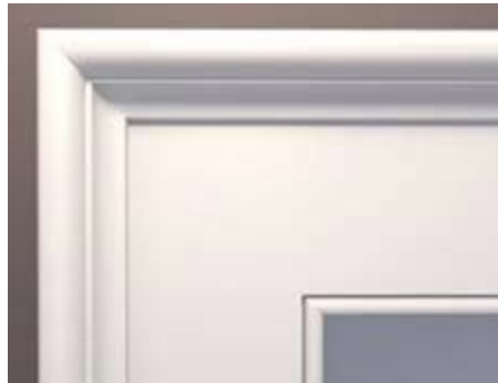
Figure 77: J-channel resembles a traditional “back band” trim when matching the trim color rather than the siding color.
